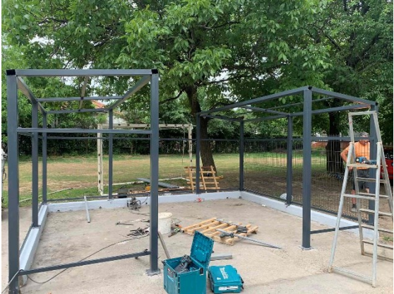
Preparation of the pilot project location
